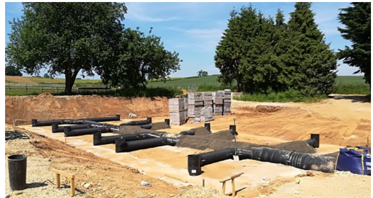
Ductwork installed before concrete foundation laid
