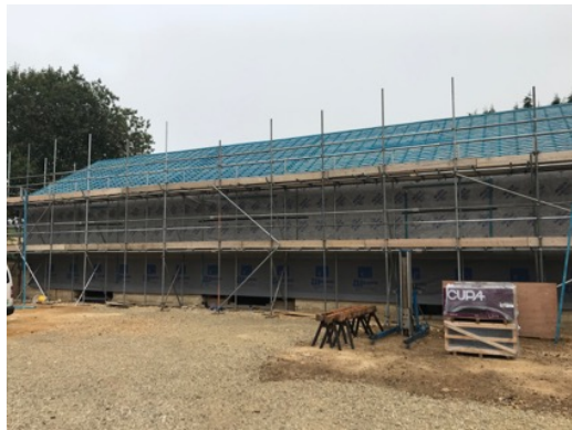
Mickleton Hills under construction
