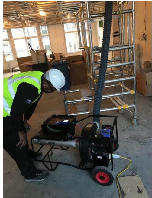
Pressure testing with PANDA 341
